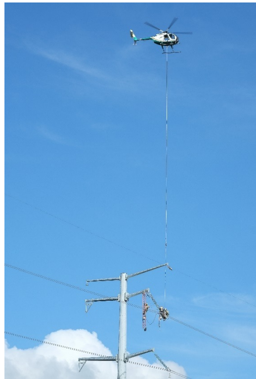
Figure 10: Helicopter installing transmission line and conductor; courtesy of Xcel Energy.
