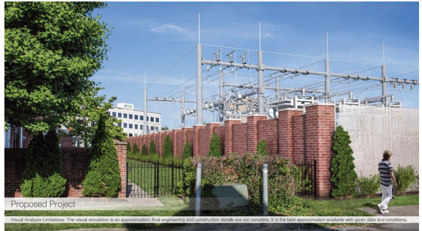
Figure 2 (top): Substation design to match neighborhood character; courtesy of AEP.
