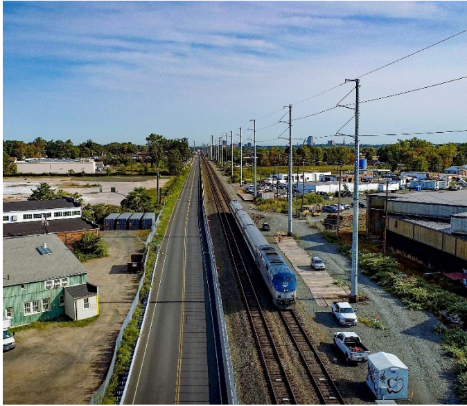
Figure 6: Overhead transmission segment on the Amtrak ROW; courtesy of Eversource.
