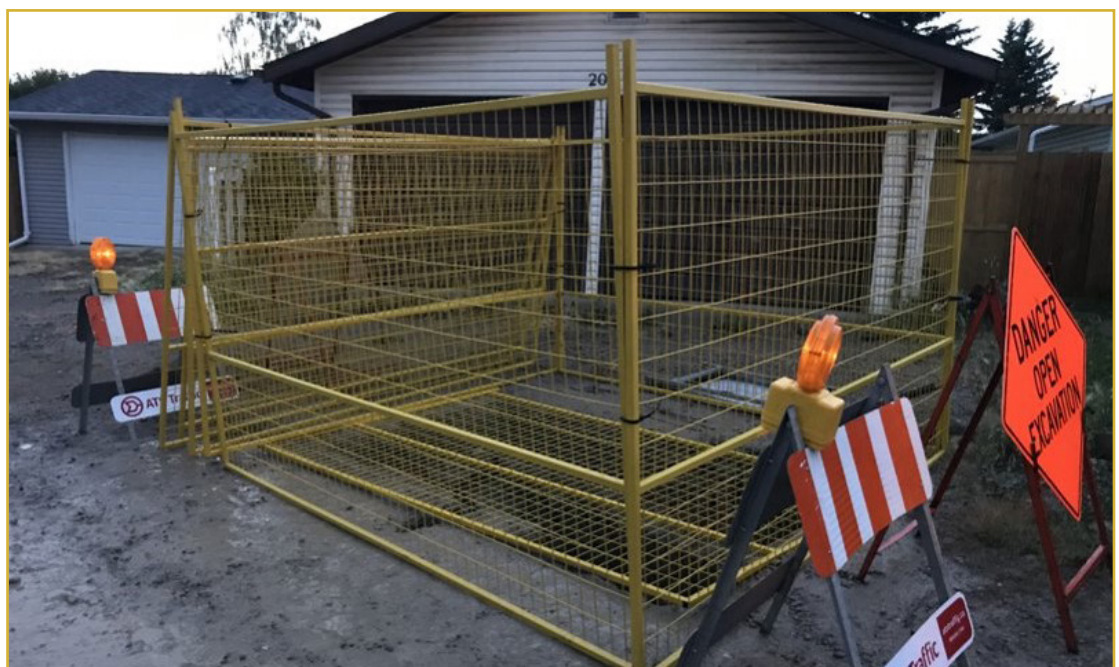
Example Cable Fault Repair Site
