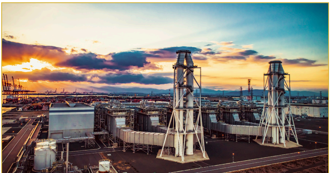
Nishi-Nagoya Thermal Power Station
